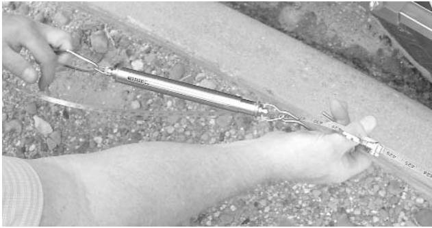
Figure 18. Using the tape tensioning device
